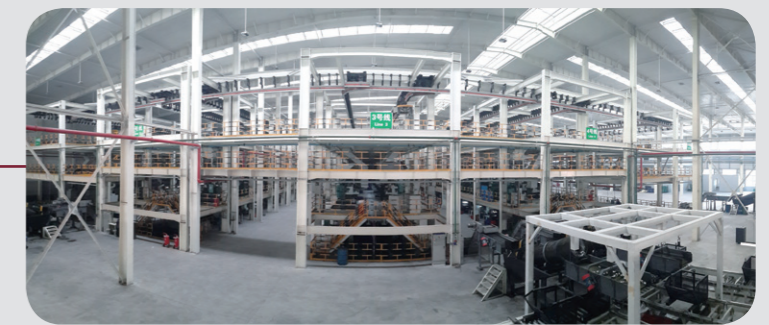
Threading, Air Pressure Test, and Anti-rust Treatment
